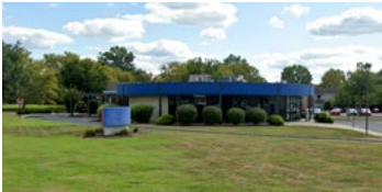
PNC BANK East Windsor, NJ
