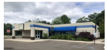
FULTON BANK Sewell, NJ
