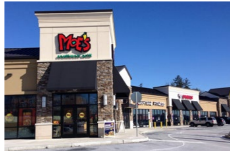
Oaks Shopping Center, Oaks, PA
